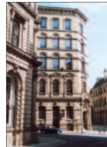
Above: Pace plc Headquarters, Saltaire
